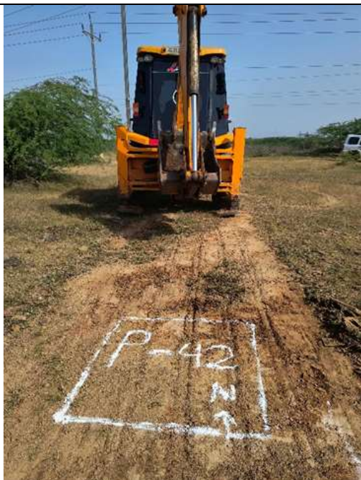
Photo. 10.2 Photograph showing the layout marking and north orientation of Pit No- 42 near Valka Nana village, prior to excavation.
